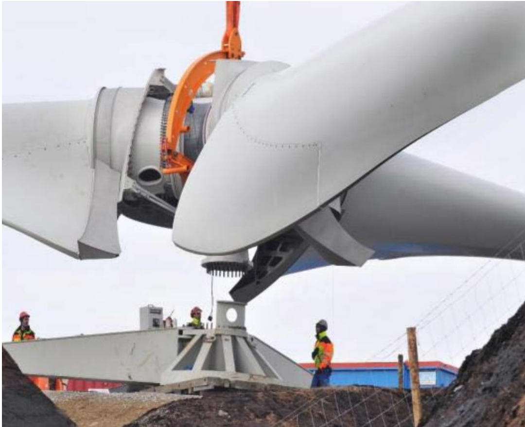
Plate 3.4: Assembly of wind turbine blades 2
