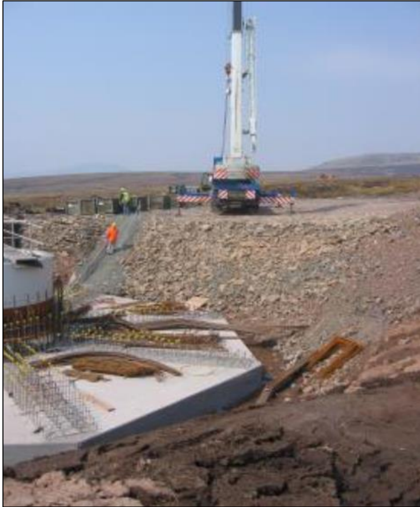
Plate 3.1: Turbine foundation under construction with adjoining crane pad 6
