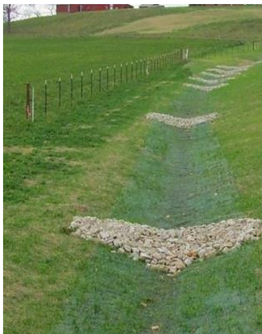
Plate 5.3: Photograph of Check Dams
