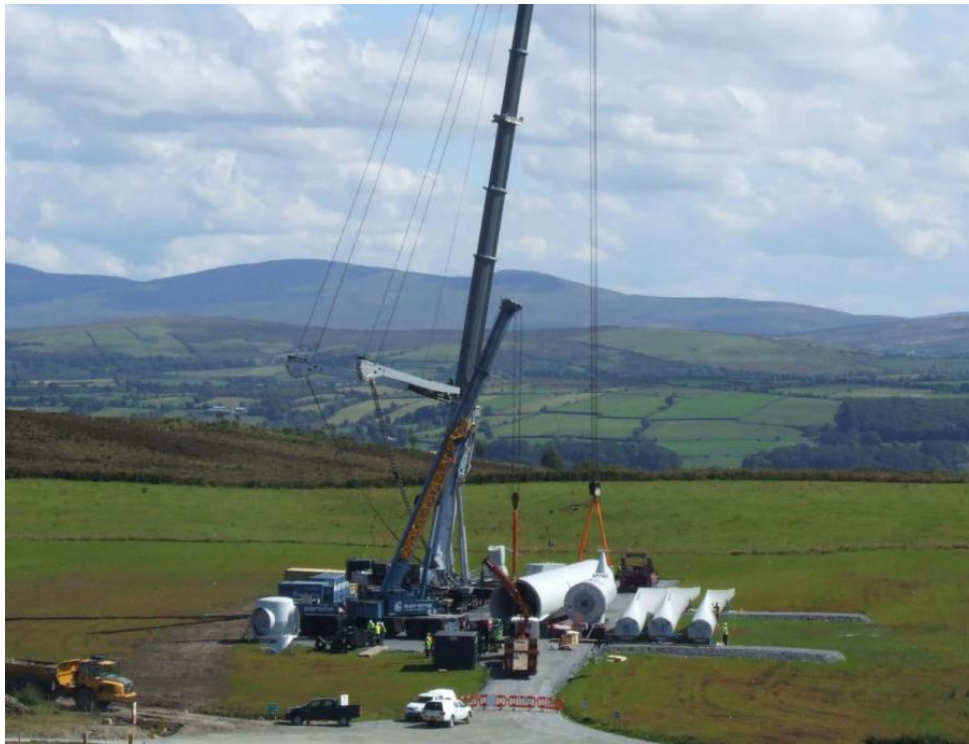
Plate 3.3: Wind Turbine Erection 2
