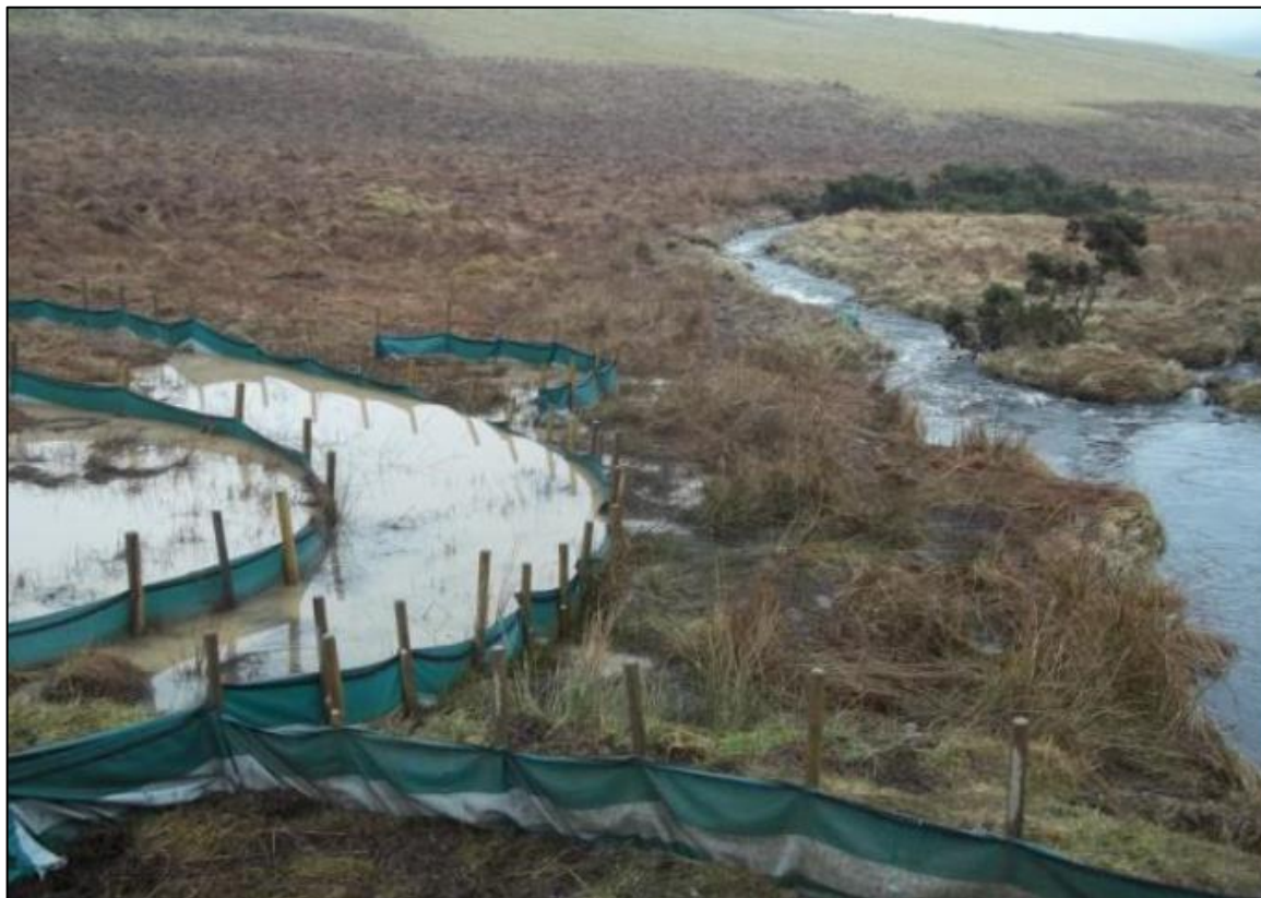
Plate 5.2: Photograph of silt fencing
