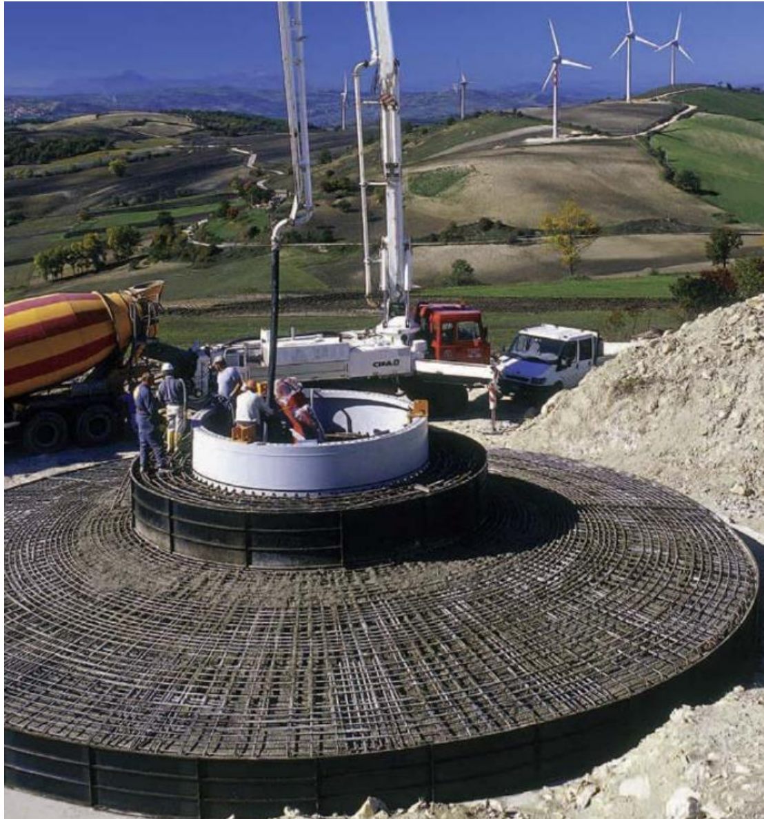
Plate 3.2: Wind turbine foundation 7
