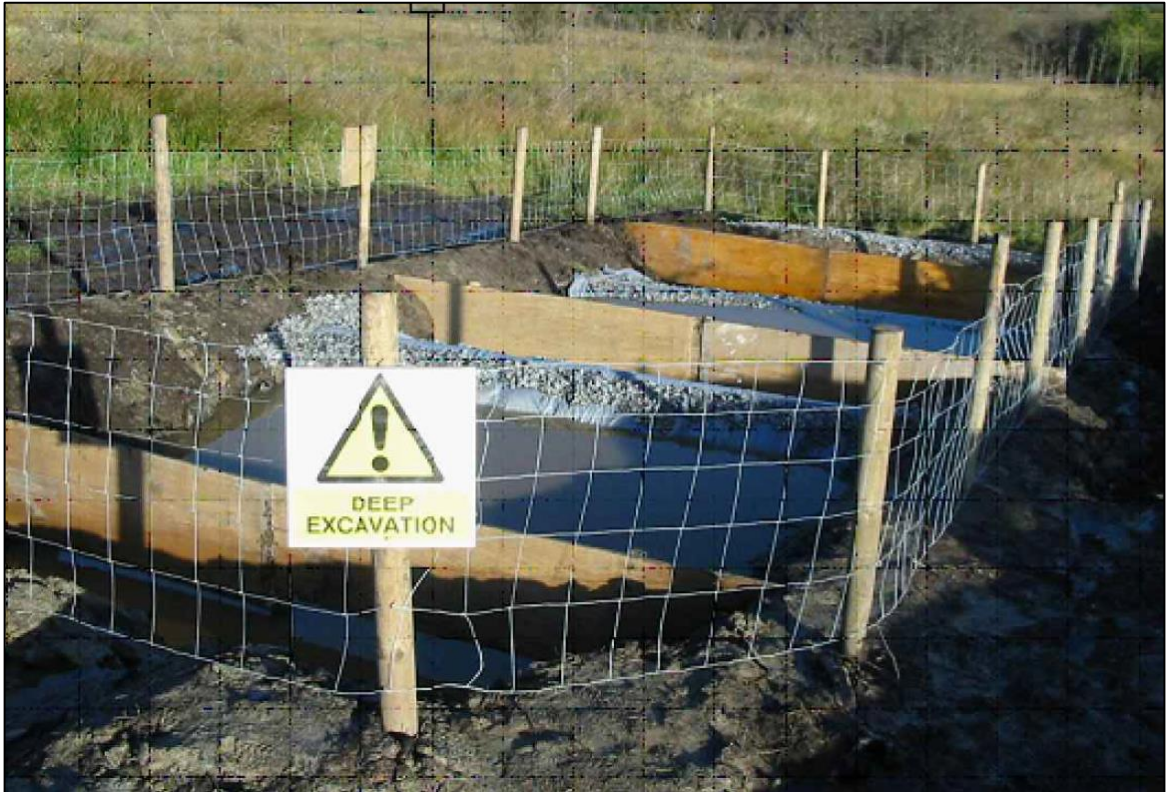
Plate 5.4a: Completed settlement pond system
