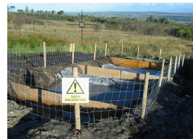
COMPLETED SETTLEMENT POND SYSTEM
